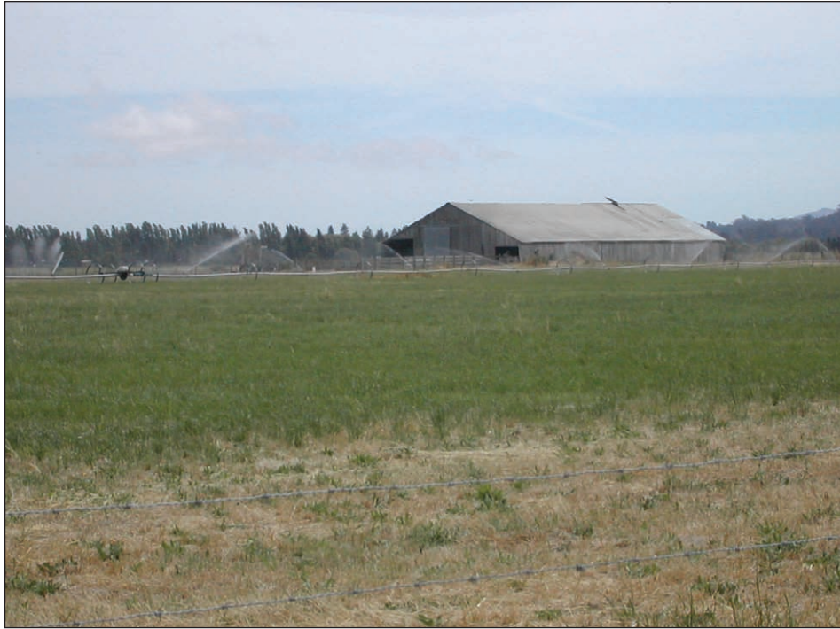
A 140-foot-long barn located near the northwest quarter of the Stony Point site. The barn has vertical board-and-batten siding with a corrugated sheet metal roof and doors. Associated with the barn is rail fencing that forms a corral and loading chute, poured concrete water troughs and a feed box for cattle.
