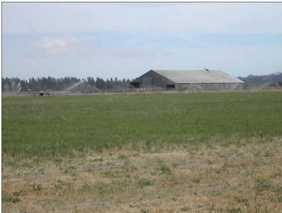
A 140-foot-long barn located near the northwest quarter of the Stony Point site. The barn has vertical board-and-batten siding with a corrugated sheet metal roof and doors. Associated with the barn is rail fencing that forms a corral and loading chute, poured concrete water troughs and a feed box for cattle.
