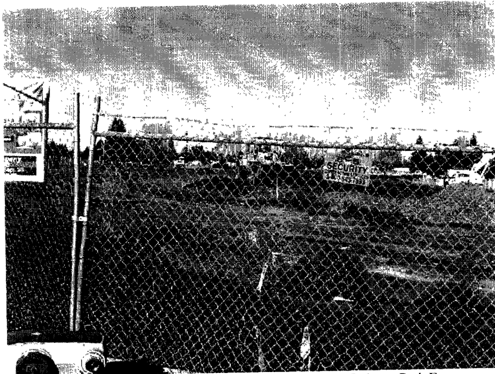
Looking west at construction at former PG&E Facility (600 Rohnert Park Expressway)
