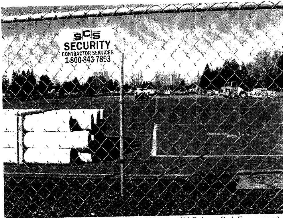
Looking west at construction on former PG&E site (600 Rohnert Park Expressway).
