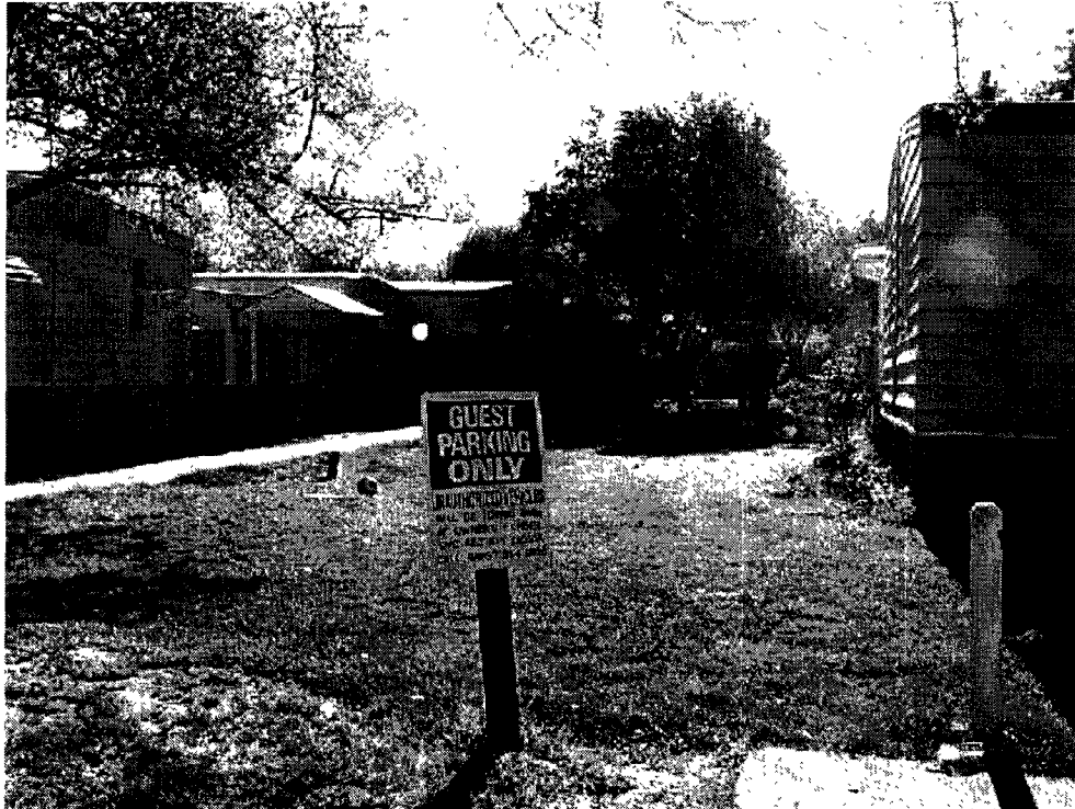
Looking southeast at Rancho Verde Mobile Home Park at the approximate location of the berm of the airplane target range.
