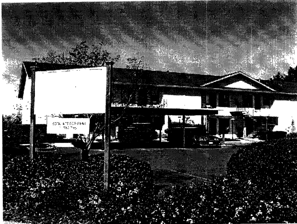
Looking west at Manor Apartments (360-458 Laguna Dr)
